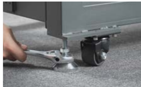
26 Tighten the four support feet to suspend all four wheels securely, securing the machine in place.
